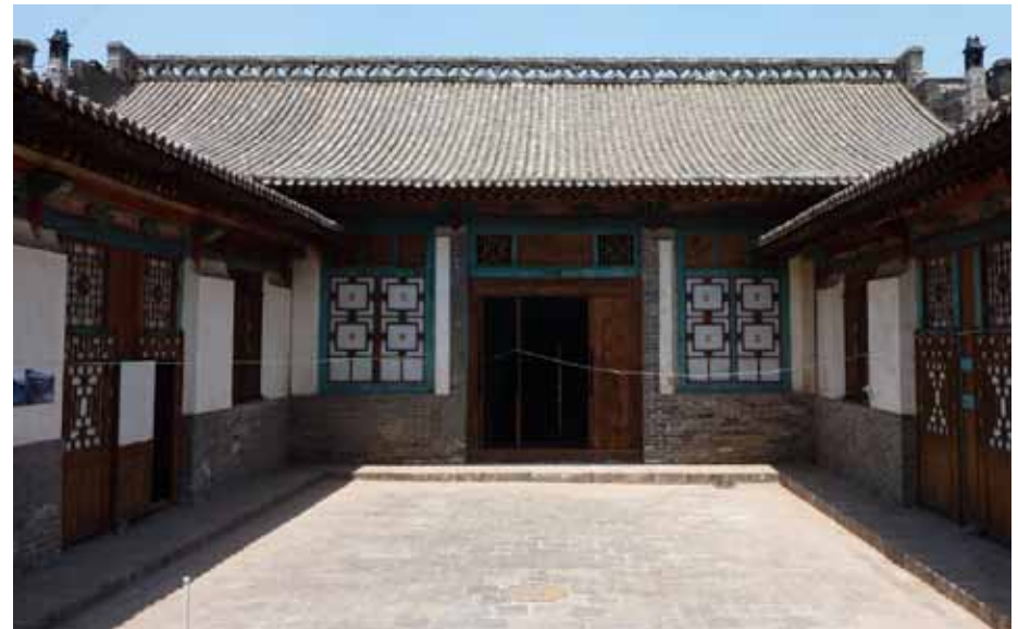
Top: Pingyao courtyard before restoration. © GHF
