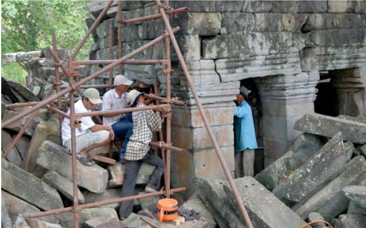
Local workers stabilizing the southeast corner of the Banteay Chhmar temple complex. Photo: GHF
