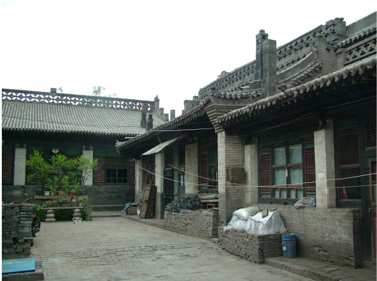
A courtyard set to be restored as part of GHF's next physical conservation project at Pingyao. Photo: Vincent Michael
