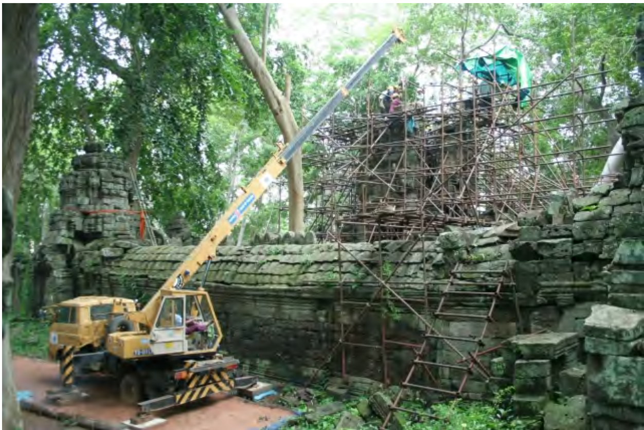
Photo: The Face Tower 18, which was heavily destabilized during heavy monsoons, receives structural support and partial disassembly with the assistance of a crane. Photo: GHF
