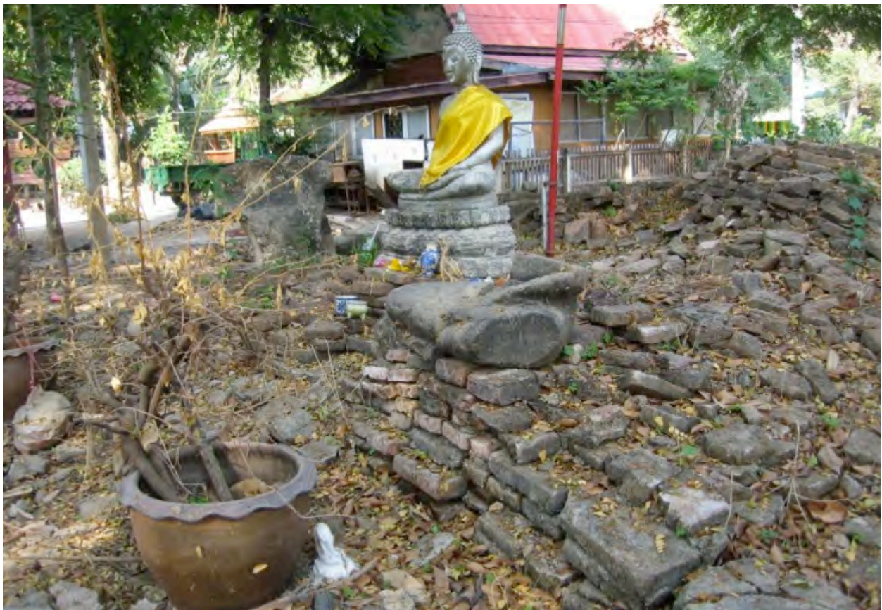
Wat Suwan Chedi shortly after receding of the October 2011 floods: Photo: GHF
