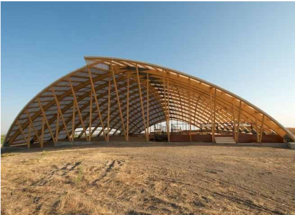
New Site Shelter, 4040 Front View. Photo by Jason Quinlan
