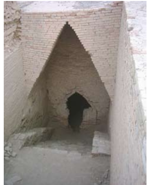
The sagging walls of the Royal Tomb entrance require support to prevent collapse. Photo by © Global Heritage Fund
